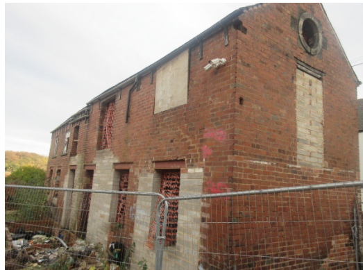
Two storey former workshop building
