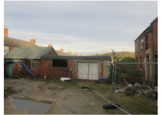
Single storey detached building
